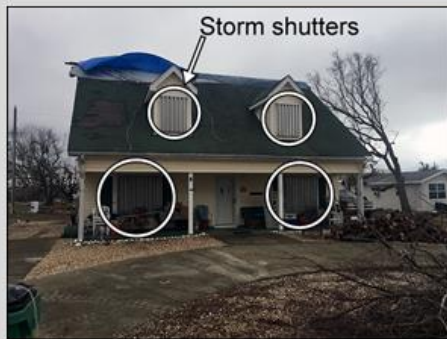
Some examples of hazard mitigation measures are house elevation, metal roofs, and storm shutters.
