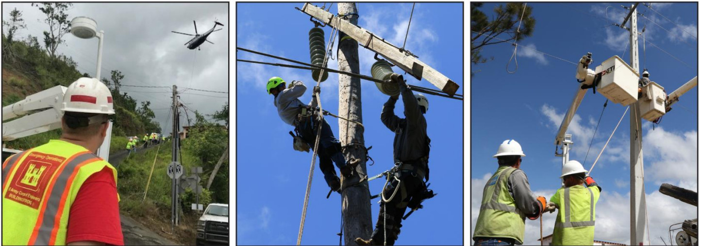
Figure 2: U.S. Army Corps of Engineers (USACE) and USACE Contractors Working to Restore Electricity in Puerto Rico
