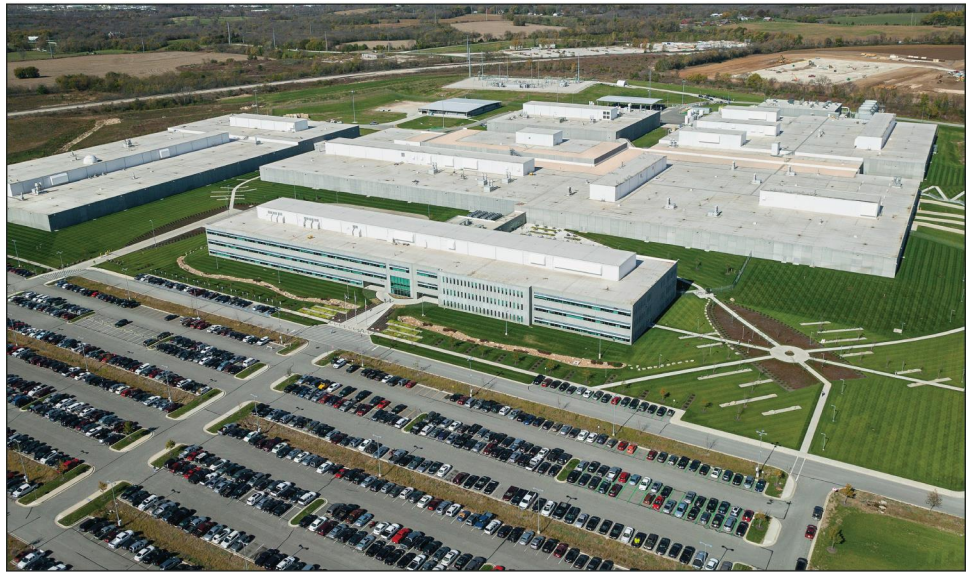
Figure 5: Photo of Kansas City Site Production Facility Built in 2012
