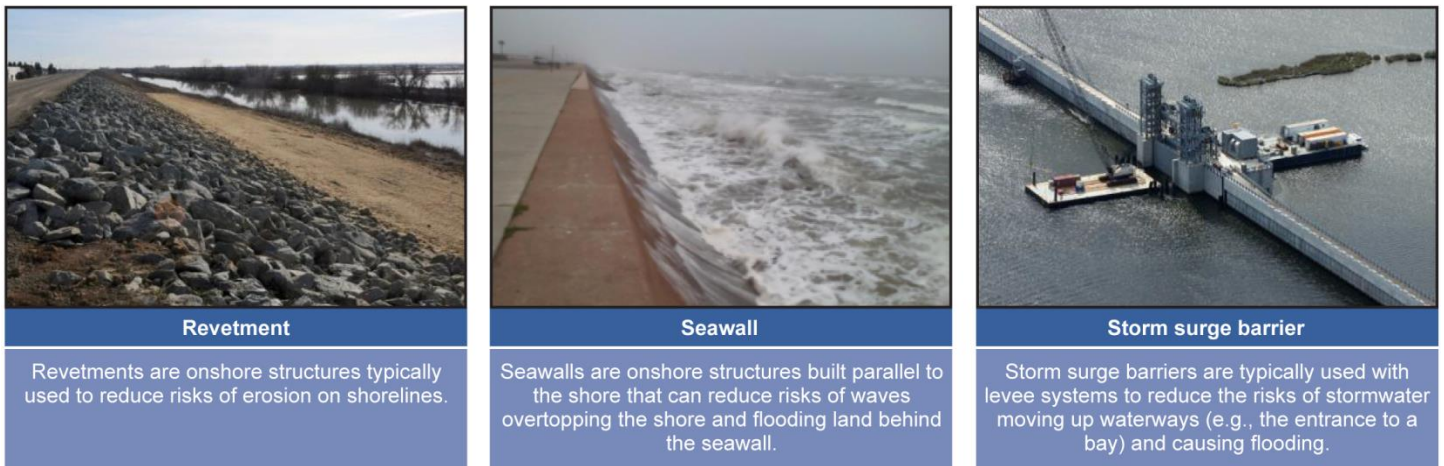
Figure 1: Examples of Hard Infrastructure the Corps May Use for Coastal Storm and Flood Risk Reduction
