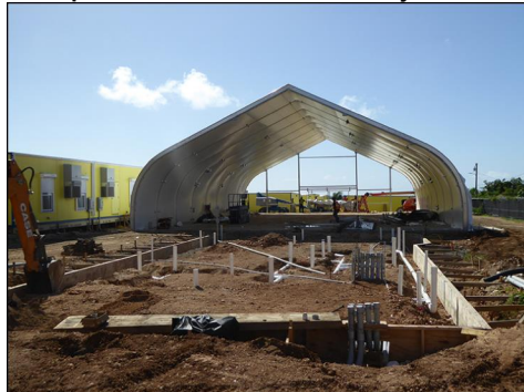
Modular units are being constructed to serve as temporary school facilities. This large unit will be the cafeteria.
