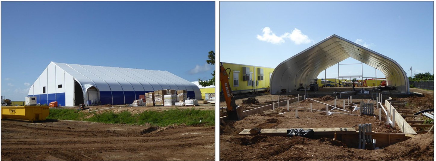
Figure 6: Construction of Temporary School Facilities in St. Croix, U.S. Virgin Islands
