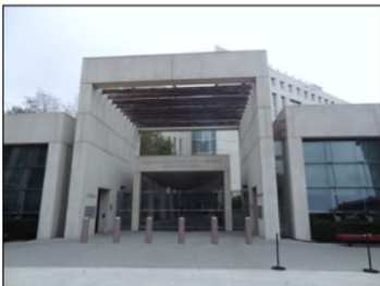
Ariel Rios Federal Building (Washington, D.C.)
