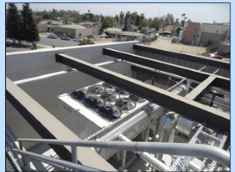
Bakersfield Federal Courthouse (Bakersfield, CA) – The mechanical systems are placed on the roof and exposed to extreme environmental conditions. Building managers have hung makeshift drapes in an attempt to protect these systems from overheating (left). Sand can clog the air intake fans for the building's air conditioning unit (right).
