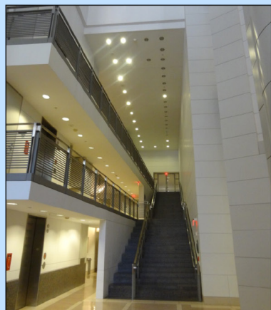
Ronald Reagan Building and International Trade Center (Washington, D.C.) – Lights over staircases are difficult to replace and require special equipment, such as scaffolds.
