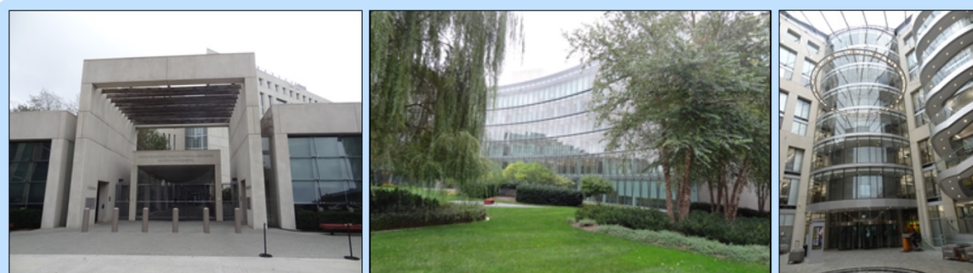
Ariel Rios Federal Building (Washington, D.C.) – Main entrance, interior courtyard, and interior atrium (from left to right).
