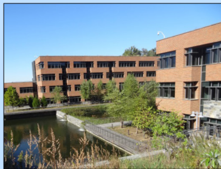
Douglas A. Munro Coast Guard Headquarters Building (Washington D.C.) – The building façades incorporate multiple materials, including two types of stone (left), brick (right), and glass and steel (bottom), which are difficult to clean. Some sections require additional equipment, leading to expensive cleaning costs.
