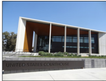
Bakersfield Federal Courthouse (Bakersfield, CA)
