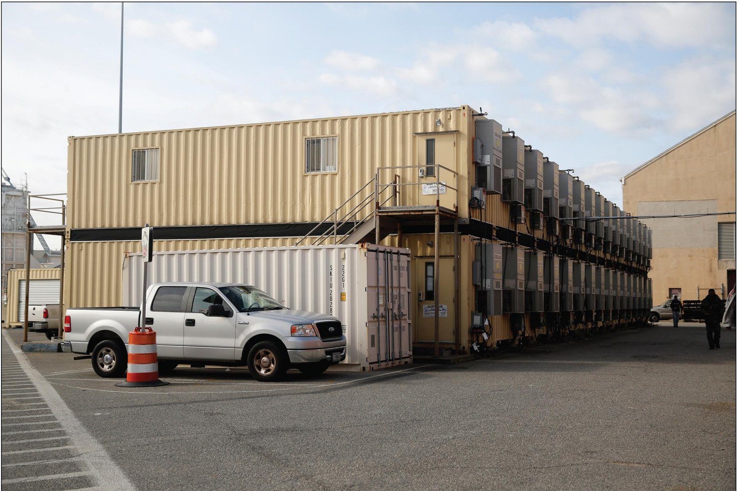
Figure 8: Double-Stacked Temporary Office Facilities at Norfolk Naval Shipyard, October 2016
