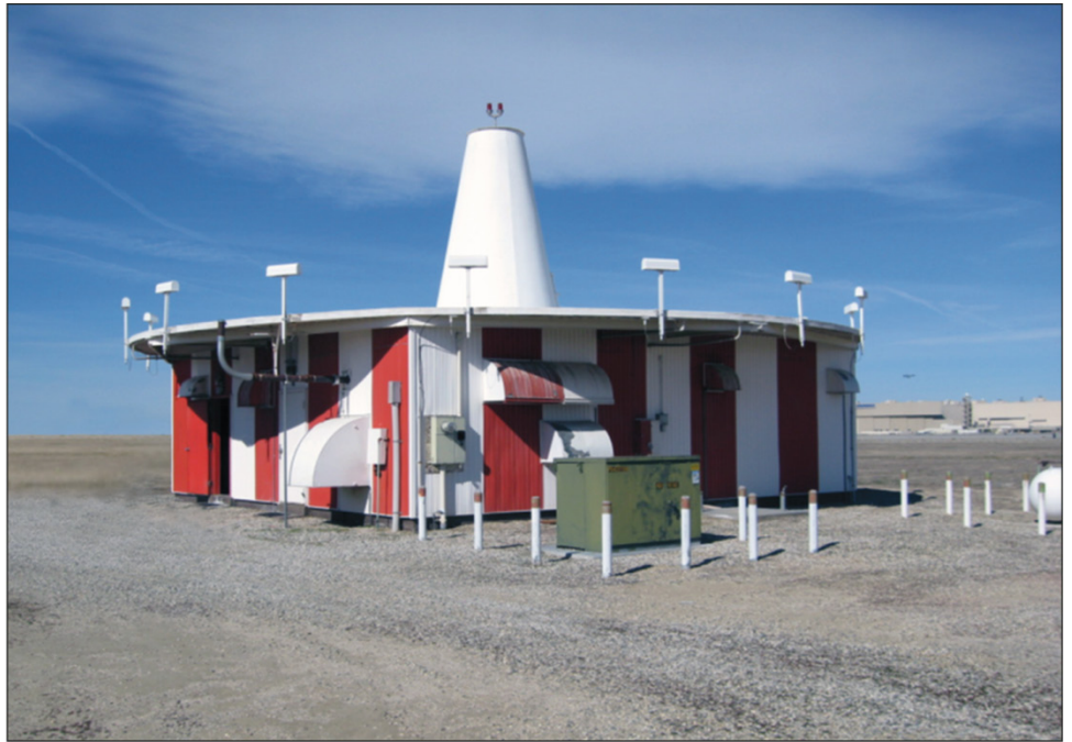
Figure 5: Very High Frequency Omnidirectional Radio Range (VOR) Station
