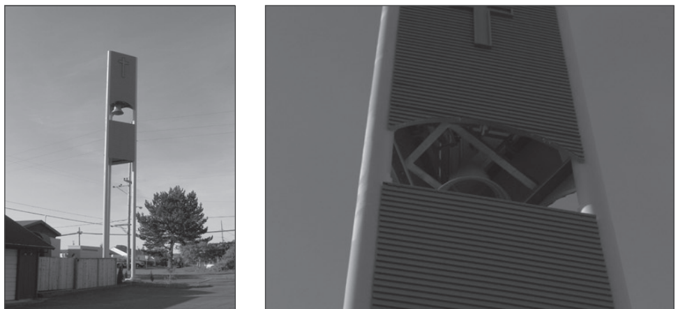
Figure 14: Disguised Cellular Tower in Eureka, California
