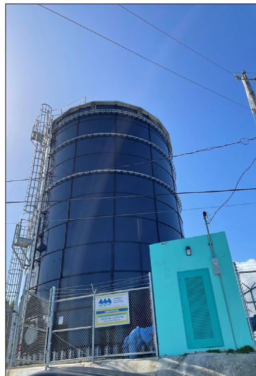
Largely repaired water tank observed in March 2022
