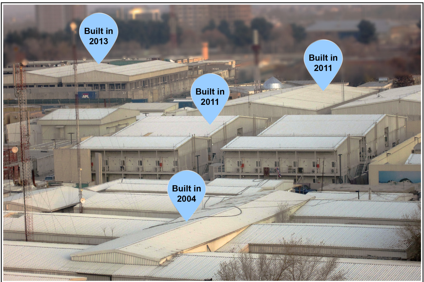
Figure 3: U.S. Embassy Kabul, Temporary Facilities
