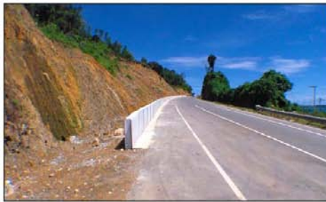
Rock-fall retaining wall
