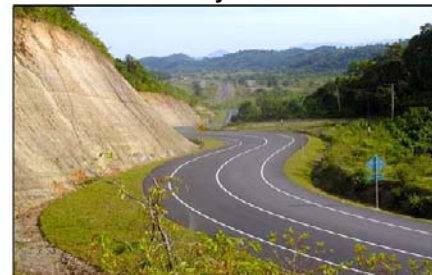
Section of new road built by USAID
