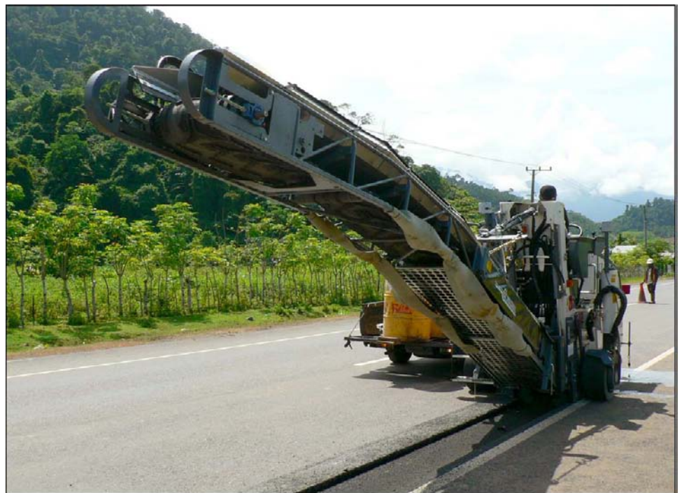
Figure 9: Milling Machine Removing Faulty Pavement in Indonesia Road
