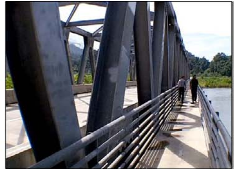
Source: GAO. Bridge walkway
