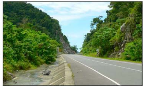
Concrete-lined drainage channel
