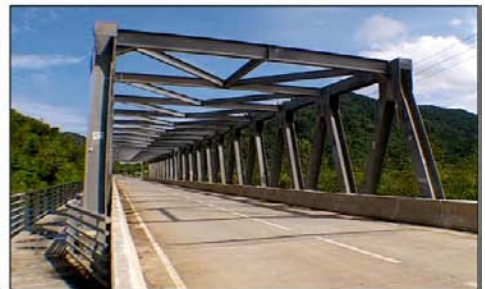
Galvanized steel bridge
