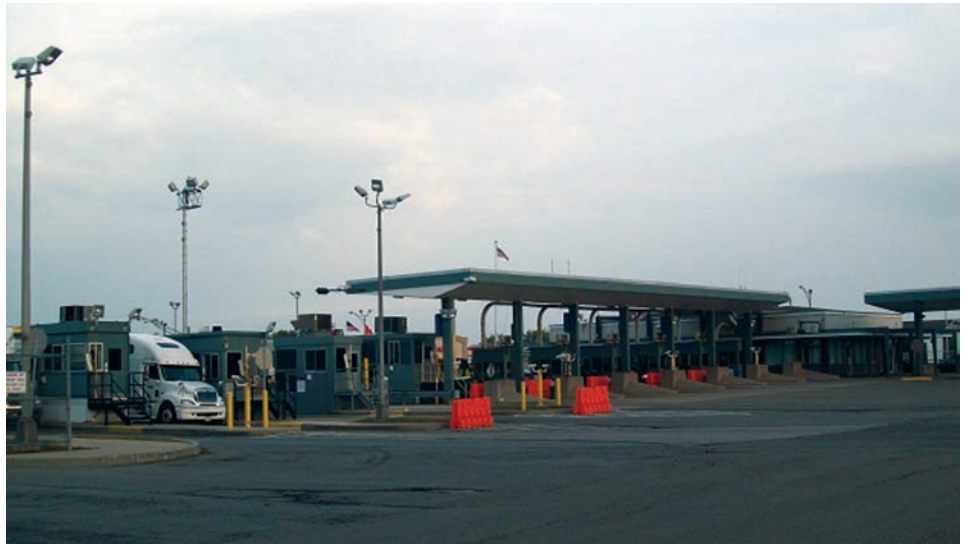
Figure 1: Lewiston-Queenston Border Crossing, Lewiston, New York
