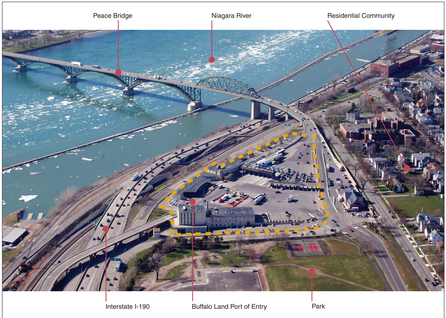
Figure 14: Overhead View of Peace Bridge Facility in Buffalo, New York
