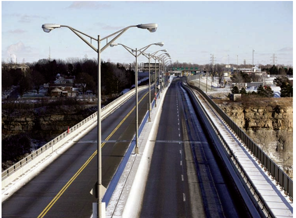
Figure 9: Lewiston-Queenston Bridge with Four Lanes Prior to Expansion Project
