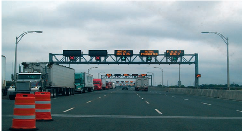
Figure 10: Lewiston-Queenston Bridge with Five Lanes after Expansion Project
