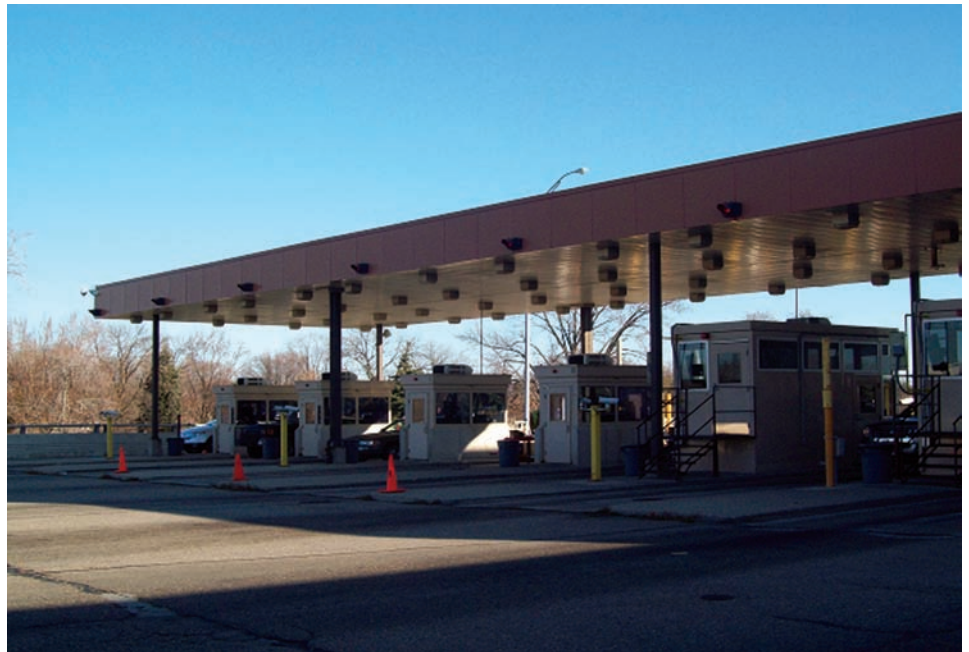
Figure 8: High-Low Processing Booth for Either Cars or Trucks Next to Four Regular Car Booths at the Port Huron Facility
