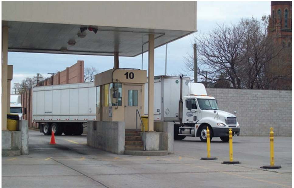
Figure 12: Truck Curving around Wall and Lane 10 to Access FAST Booths Ahead
