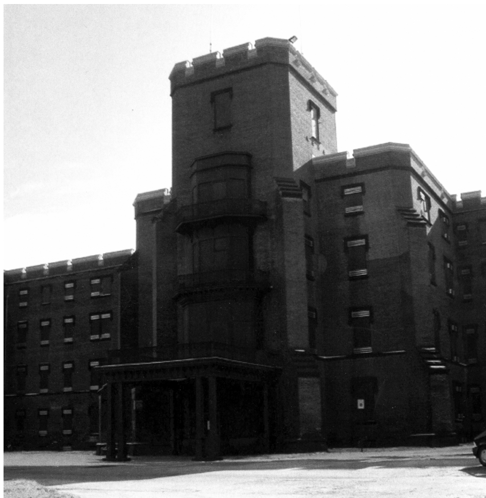
Figure 2: The Vacant Center Building, St. Elizabeths Hospital, District of Columbia
