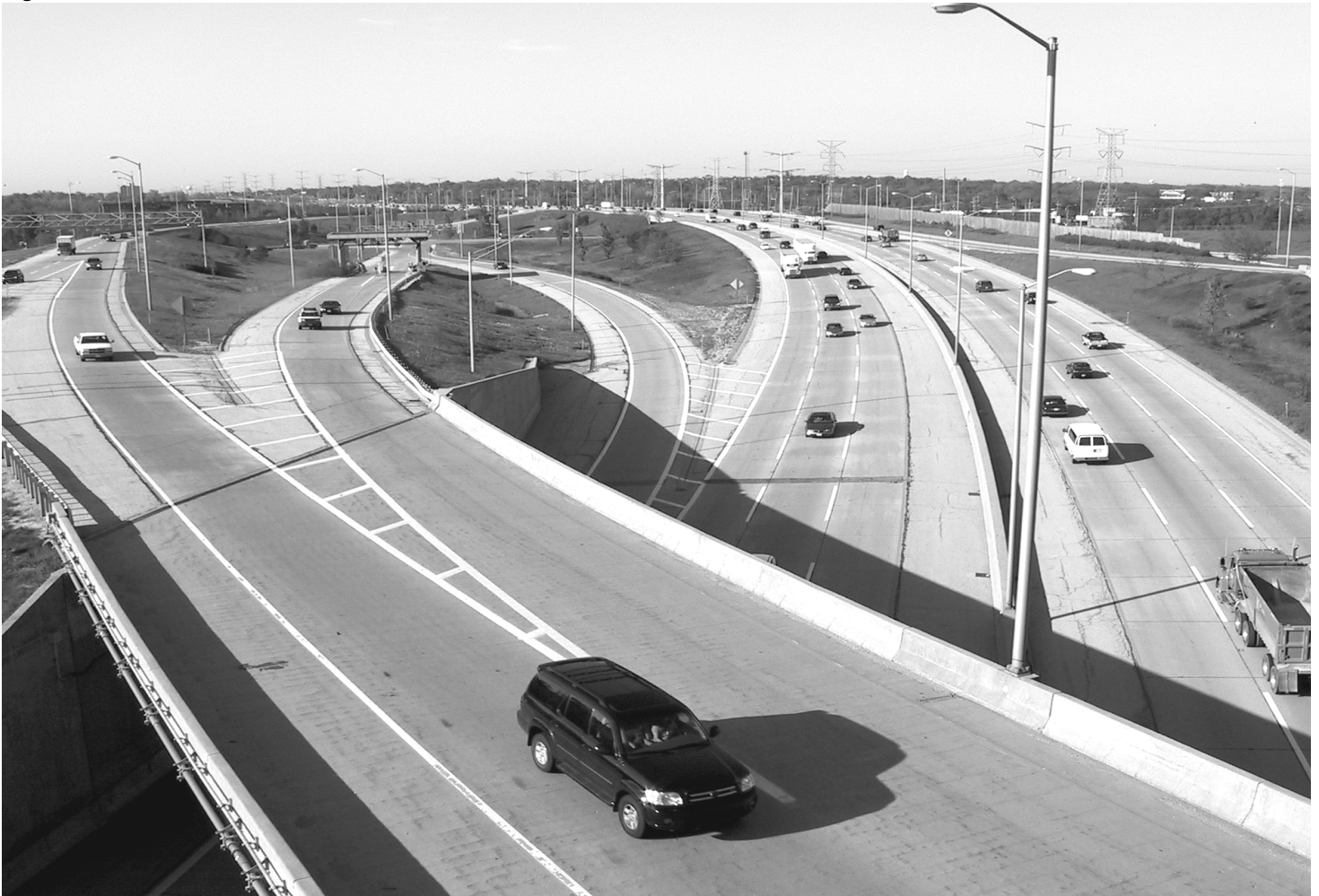
Figure 2: Overview of Interstate Section
