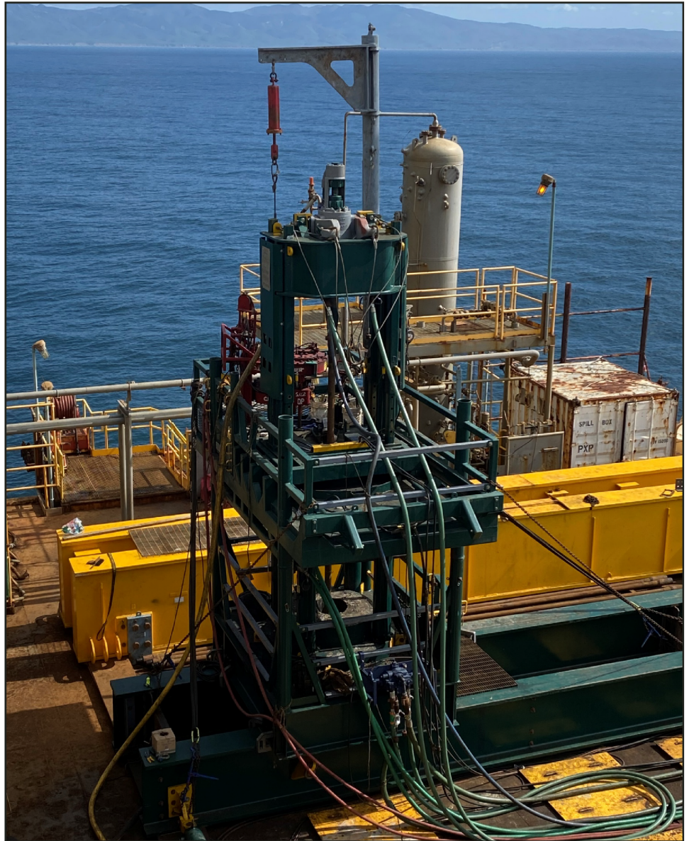
Figure 6: Offshore Well Plugging Operations in the Pacific Region
