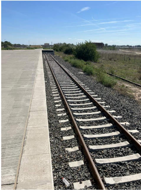
Figure 6: Railhead at Mihail Kogălniceanu Air Base, Romania
