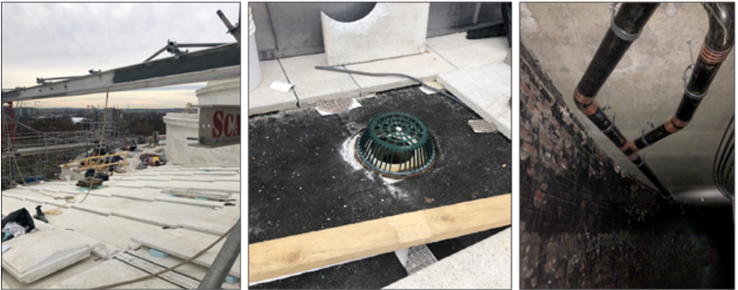
Figure 2: Project at the Jefferson Memorial That Sealed Roof Tiles, Added Drains, and Installed Pipes (left to right) to Address Precipitation Risks
