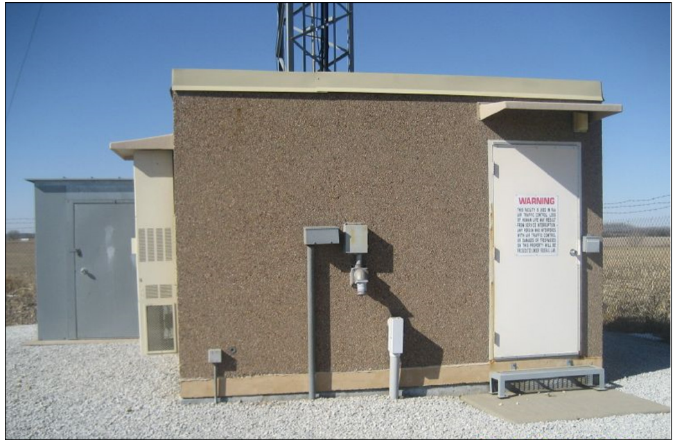
Figure 5: An Excess FAA Building Located on Airport Property
