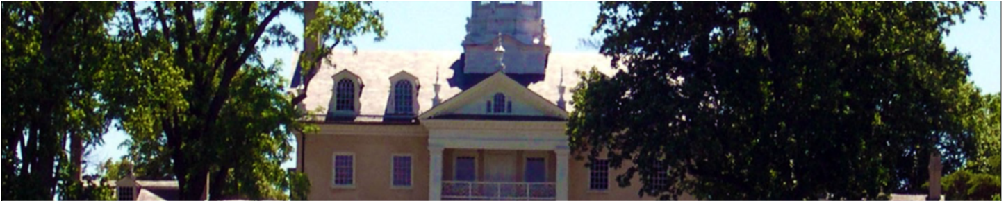
Figure 17: Hampton National Historic Site
