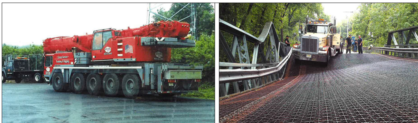
Self-propelled 170,500 pound crane traversing the bridge when it collapsed
