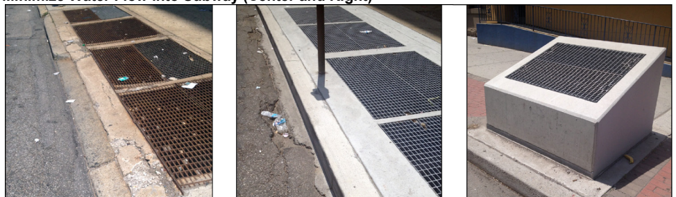
Deteriorated Curb Allowed Water to Flow in Subway (Left) and Raised Curb and Vent That Minimize Water Flow into Subway (Center and Right)
