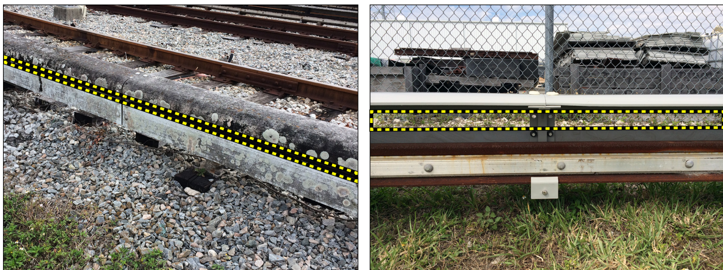
Figure 5: Miami-Dade Transit's Cover Boards for the Third Rail: Old Design Can Be Blown Off by High Winds (Left), and New Design Mitigates Wind Damage (Right)
