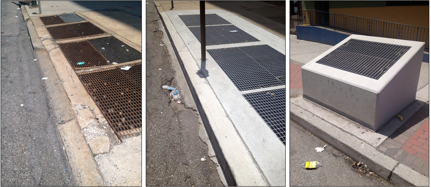
Figure 6: Deteriorated Curb That Allowed Water to Easily Enter Subway (Left) and Raised Curb and Vent That Minimized Water Flow into Subway (Center and Right)
