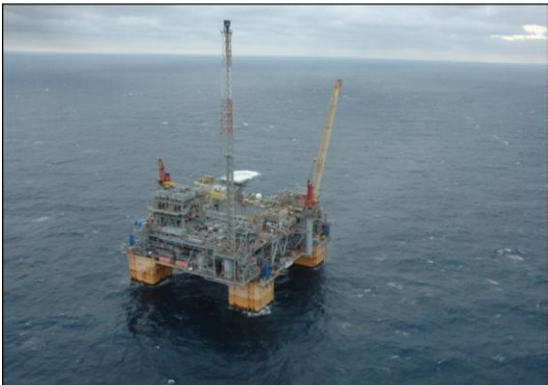
Drilling platform (near coastal)
