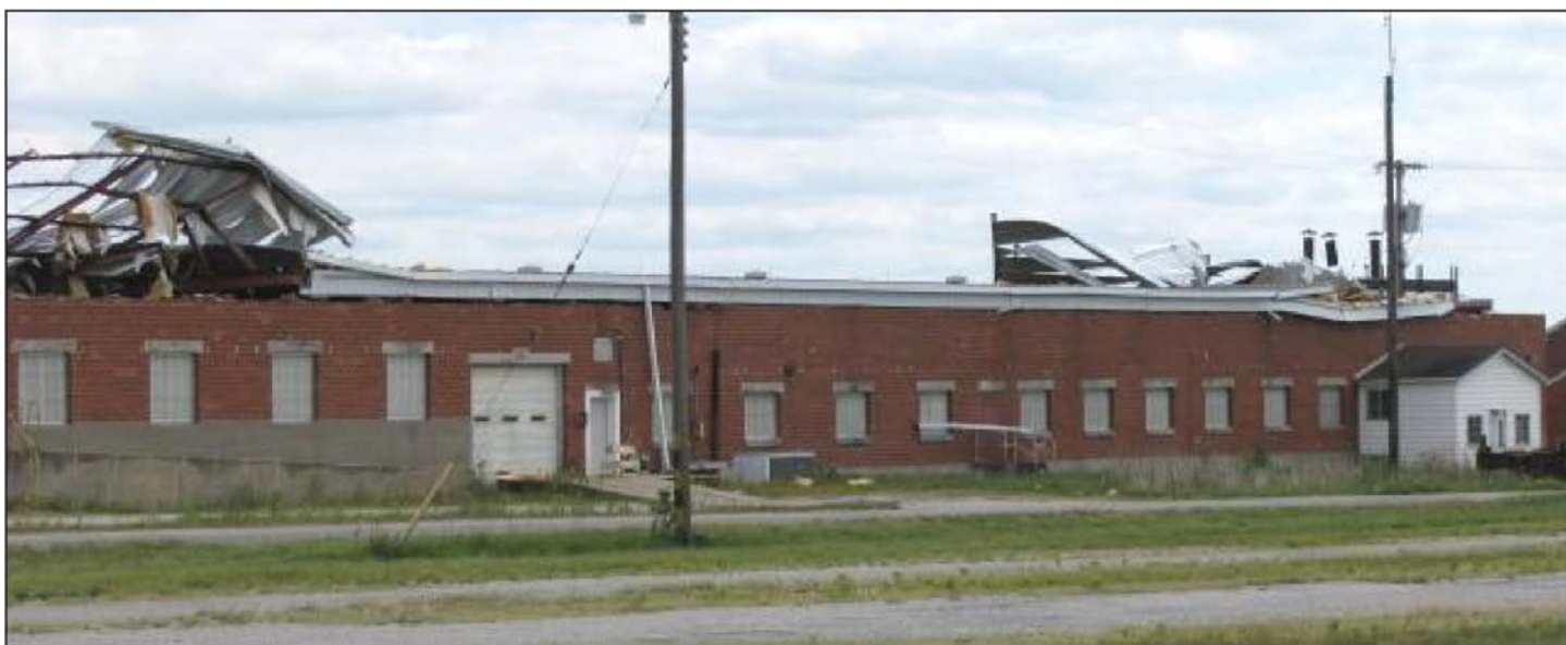
Figure 7: Damaged Roof at Kansas Army Ammunition Plant
