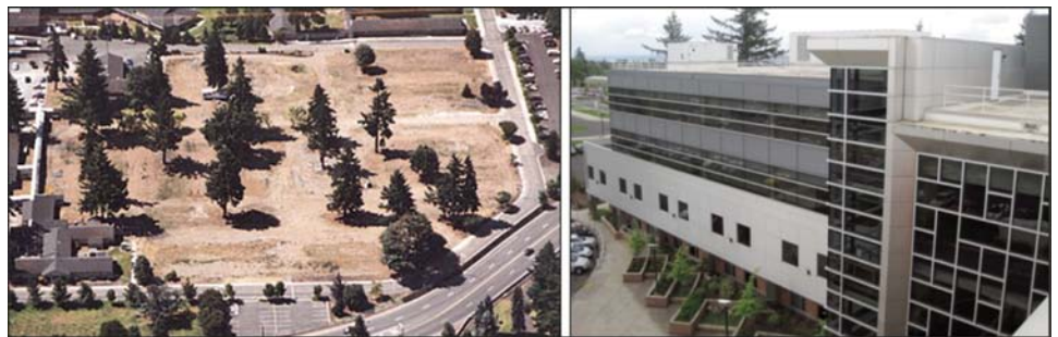
Sources: Swinerton Builders (left) and GAO (right).
