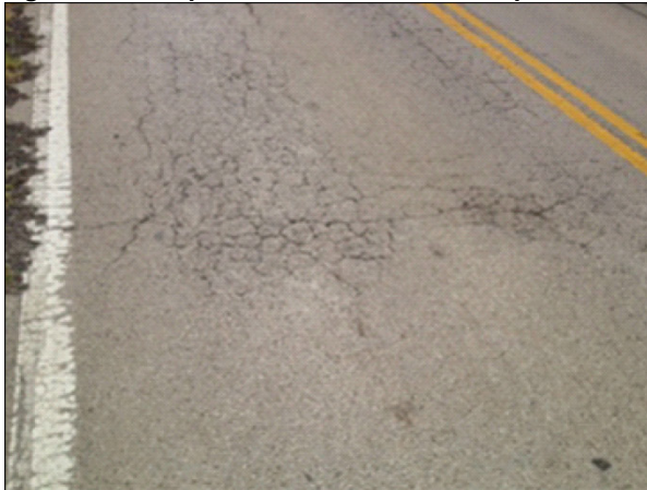
Alligator cracking of asphalt pavement.
