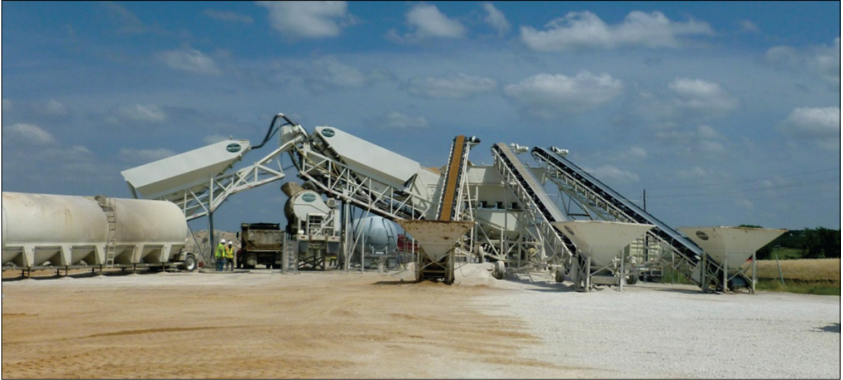
Figure 4: Concrete Plant Producing Optimized Aggregate Concrete for the Highways for Life Project in Tarrant County, Texas, 2012
