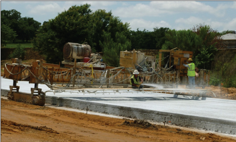
Figure 5: Application of Concrete Curing Compound at the Highways for Life Project in Tarrant County, Texas, 2012
