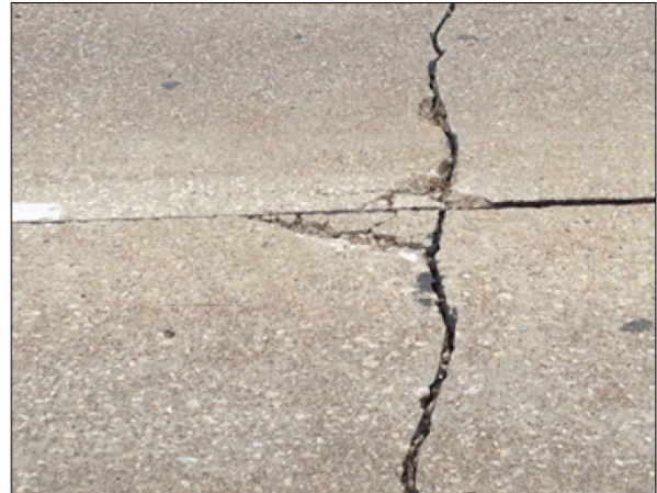
Transverse crack in concrete pavement.
