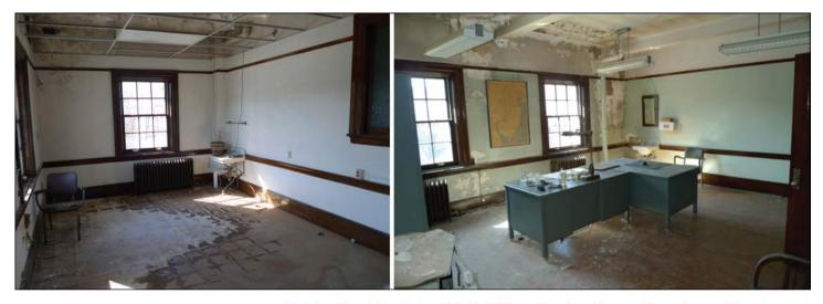
Upstairs offices in the Easton Main Post Office with walls, ceilings and floors damaged by water. Source: GAO.
