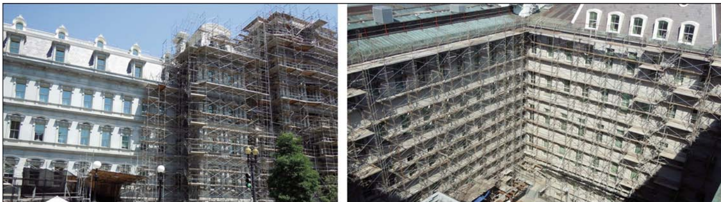
Source: GSA. Eisenhower Executive Office Building under renovation.
