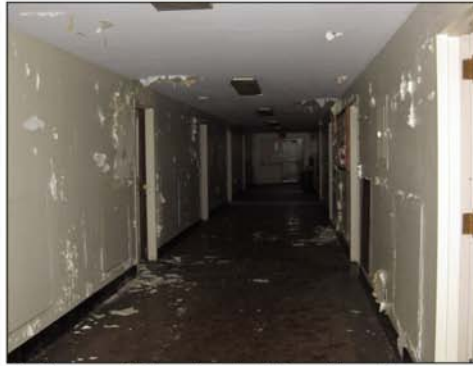
Mostly vacant laboratory building with ceiling and wall damage.
