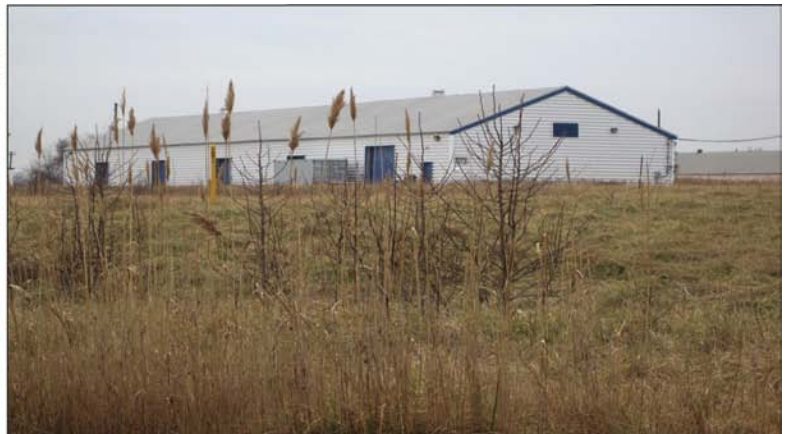
Warehouse located at GSA site.
