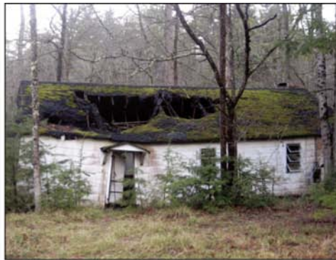
Cabin with collapsed roof.
