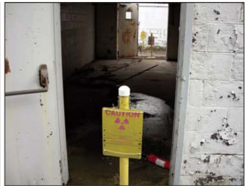
Warehouse with radiological contamination.
