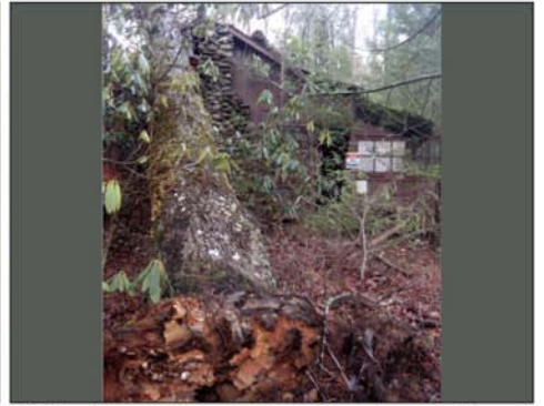
Cabin with large tree that has fallen through the roof.
