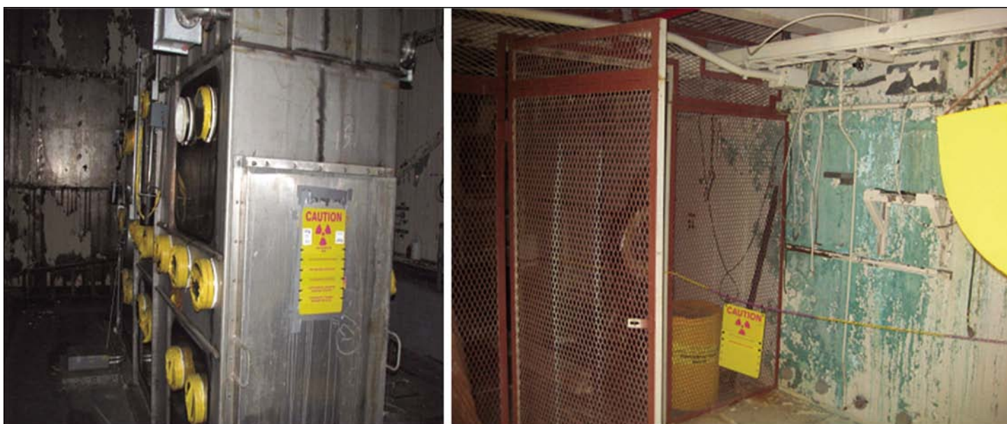
Figure 12: Vacant DOE Property with Radiological Contamination
