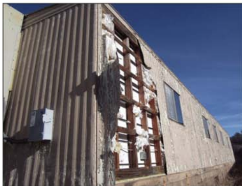
Vacant trailer with safety and health issues (rat and beehive infestation). Now demolished.
