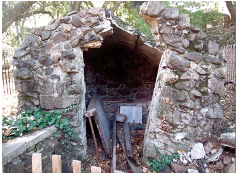
Figure 11: Interior Property No Longer Slated for Demolition because of Historic Designation Challenges
