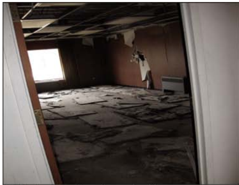
Old firehouse with collapsed ceilings.
