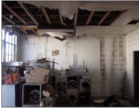
Warehouse with a collapsing ceiling.
