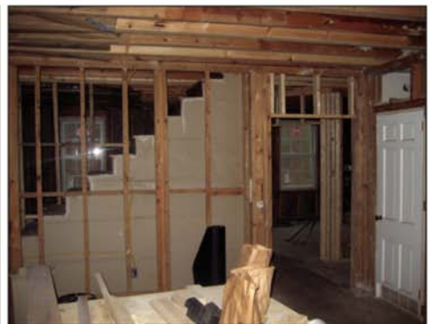
Building under renovation.
