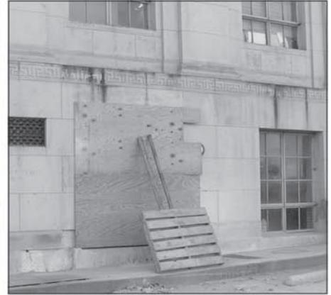
Plywood, partially secured by a wood plank, covers a broken window.
