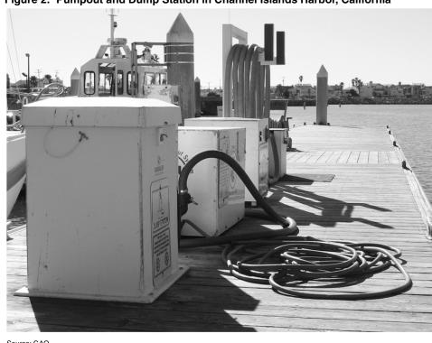
Figure 2: Pumpout and Dump Station in Channel Islands Harbor, California
