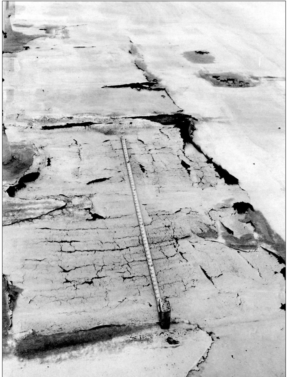
Figure 2: Roof Deterioration on the Vehicle Assembly Building at Kennedy Space Center (the tape shows a 5-foot section for perspective)
