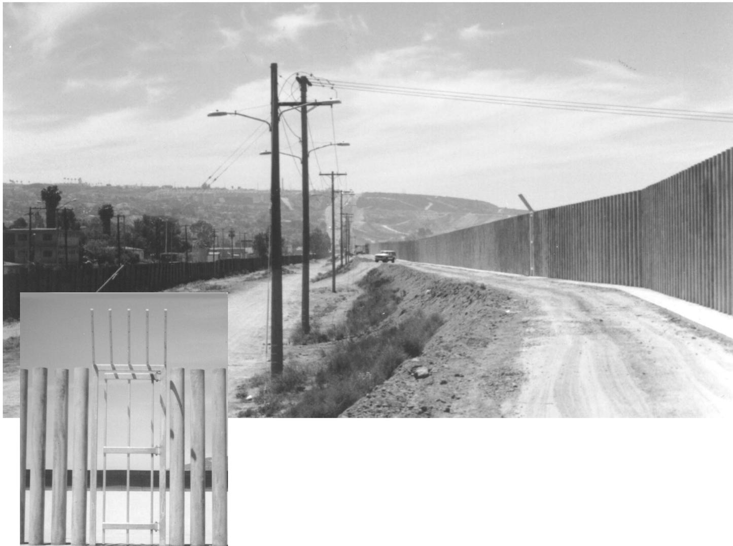
**Insert:** Bollard fencing showing electronic security access gate. Gate is to have mesh-like covering over the openings.
