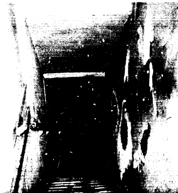
HOME INTERIOR--BROKEN HANDRAIL AND PEELING PLASTER AND PAINT.
