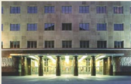
GAO headquarters building.
